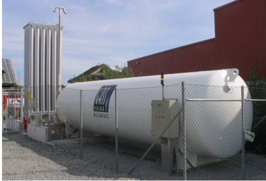
Figure 6. Small satellite plant 21 m 3 storage, 50 Sm 3 /hour
