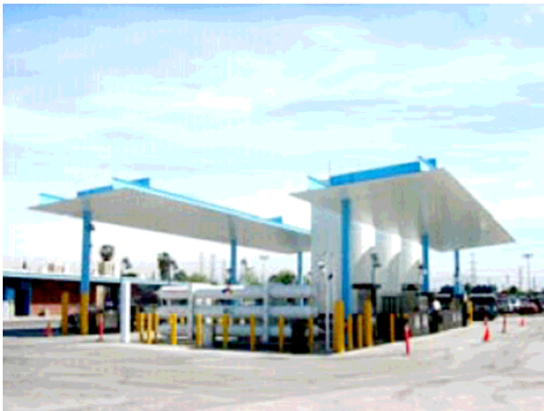
Figure 9. LNG/LCNG station, Los Angeles, CA, USA. 3 CNG dispensers, 6 LNG dispensers, serving a fleet of LNG refuse haulers and CNG-city busses.
