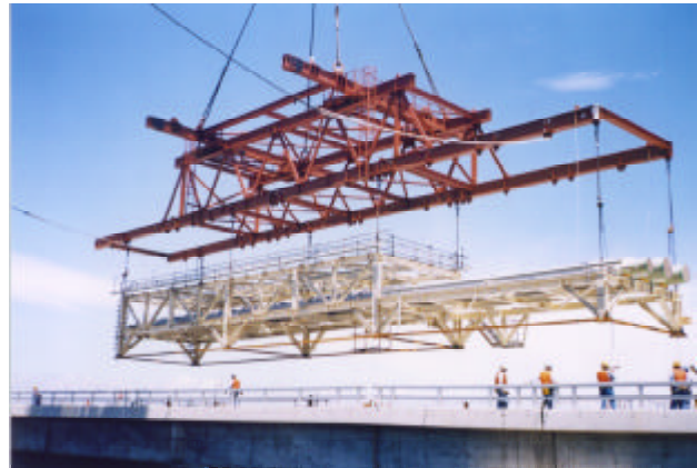
Fig.6 Unit construction method adopted for the pipe rack
